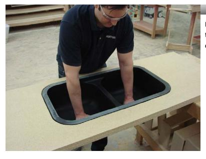
Flip the countertop over. Place the sink carefully into the opening. The sink will now be resting on the 1/2" overhanging support board.
