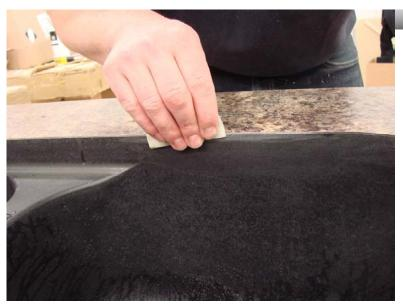
A little sanding will likely be needed to smooth the laminate edge. Use a 80 or 60 micron paper. Focus your sanding on the upper 1/4" of the bowl wall and the laminate only.
