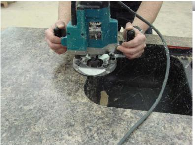
Remove the tape and adhesive drips. Lower the router bit slightly in the router and make another pass around the sink. Check how much laminate remains. If you feel you can take slightly more laminate off with the router, lower slightly then make another pass.
